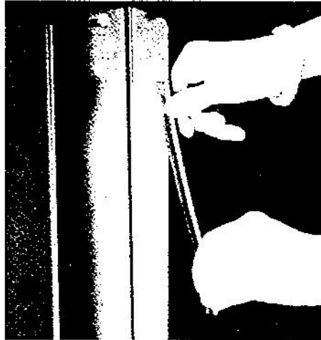
Figure 2-1: Attaching the moulding
